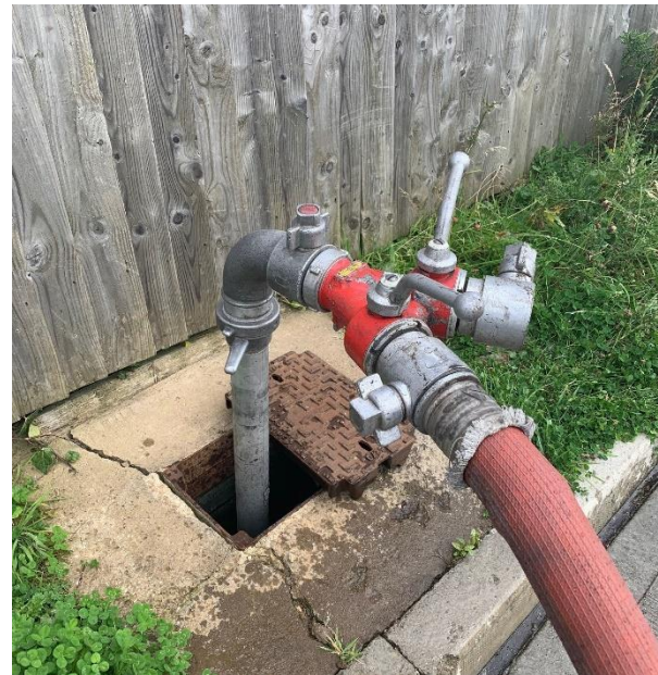
Figure 1: Working directly from a hydrant using hand controlled dividing breaching
