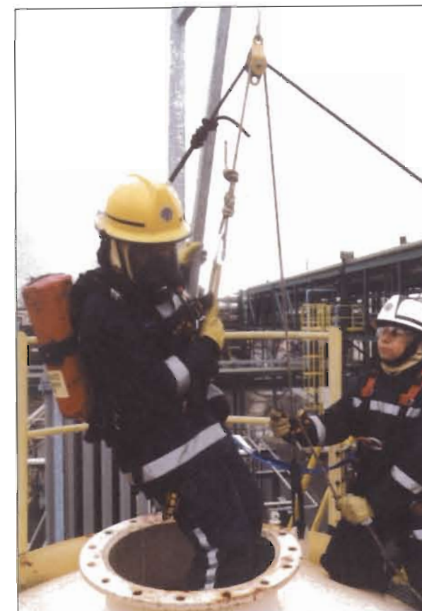
Figure 2.15 Example of a work positioning system in use above a silo.
