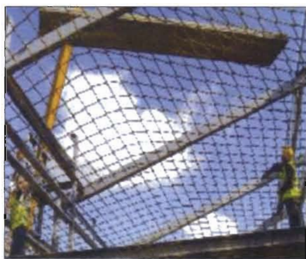
Figure 2.1 Safety nets on construction site. (Photo: Health and Safety Executive)
