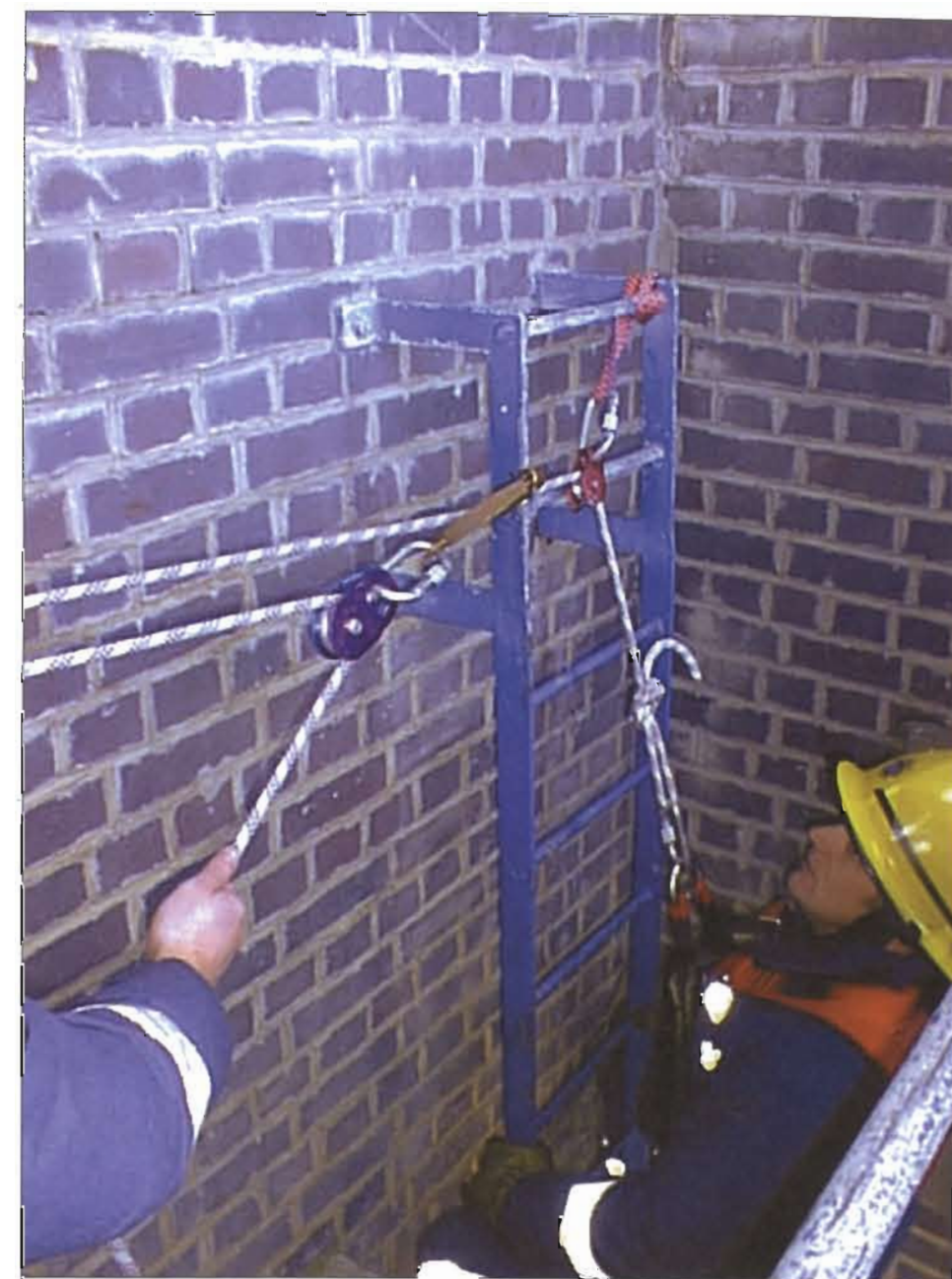
Figure 2.22 A simple 3:1 recovery system in operation.
