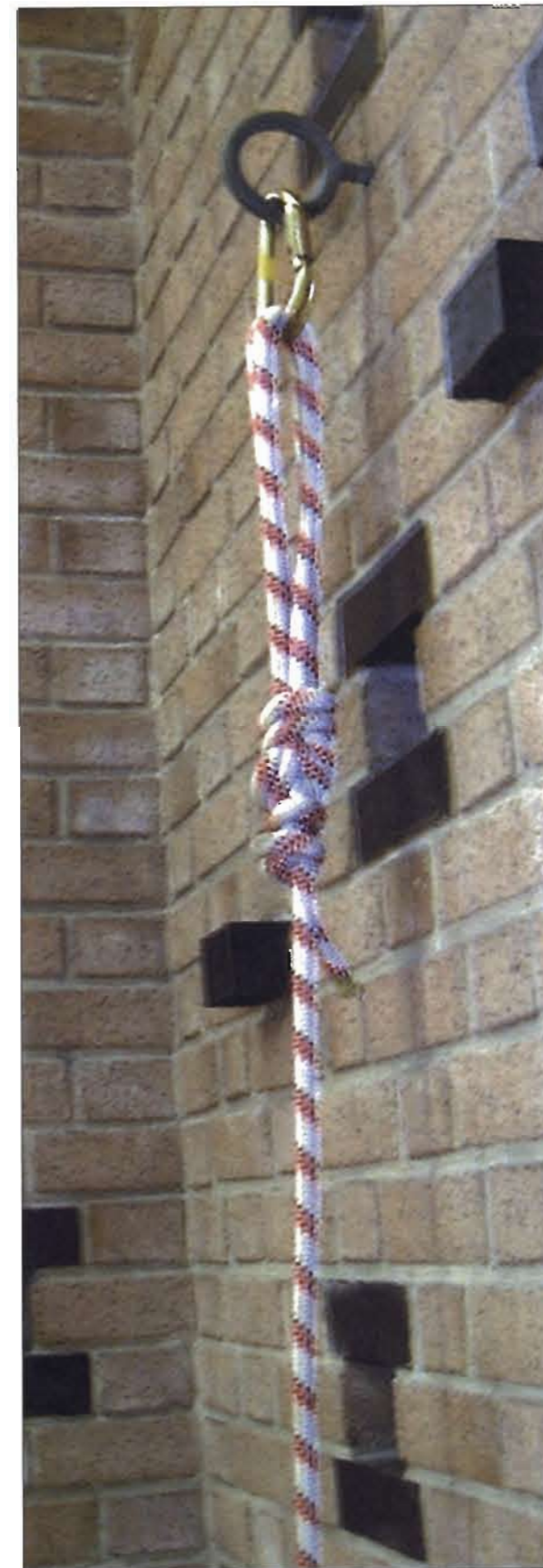
Figure 2.26 Photo of permanent artificial anchor.
