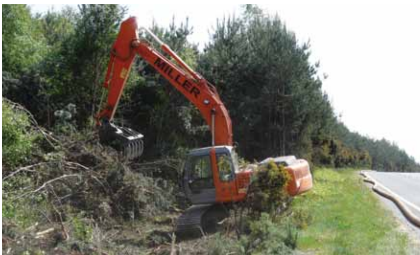
◀ Photo B8.9 Heavy machinery being used to clear scrubland
