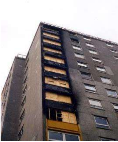
Figure: Photograph of post-fire damage illustrating the result of the Coandă effect, courtesy of the Building Research Establishment
