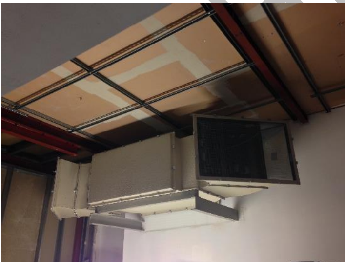
Figure 11: Smoke and heat exhaust ventilation system
