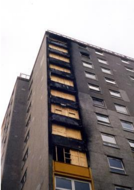
Post-fire damage illustrating the result of the Coandă effect
