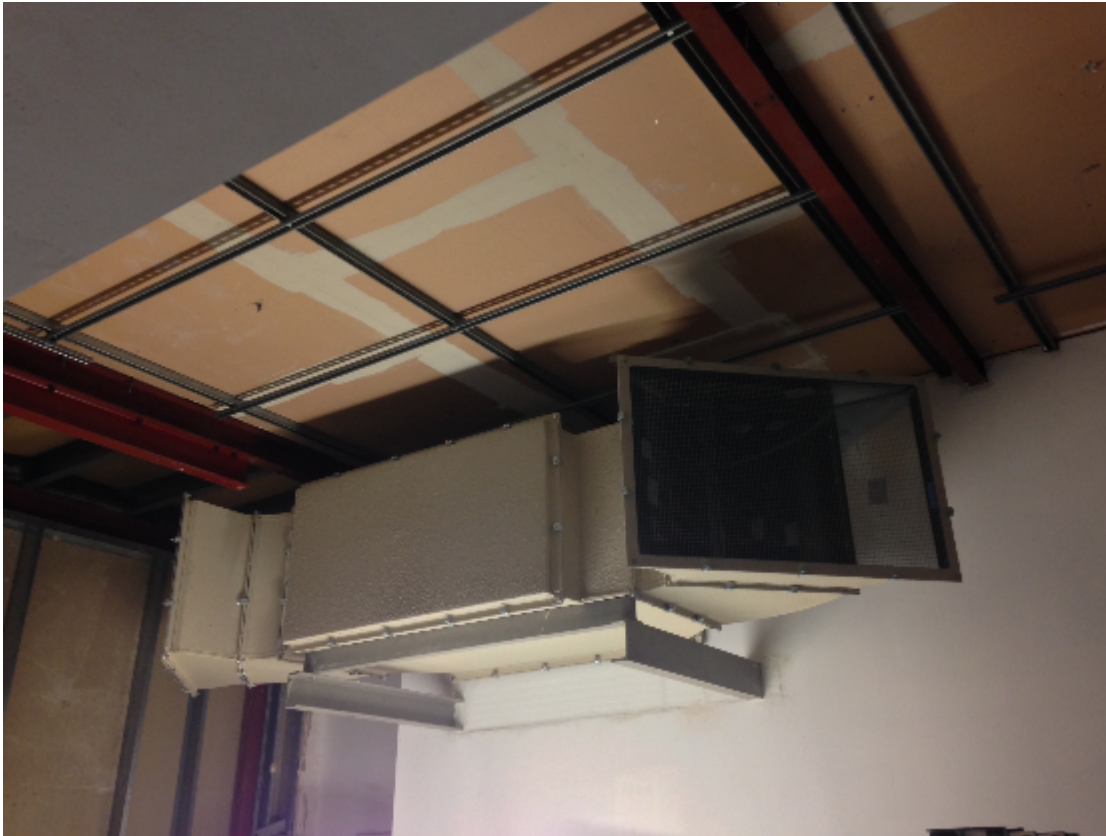
Figure 11: Smoke and heat exhaust ventilation system
