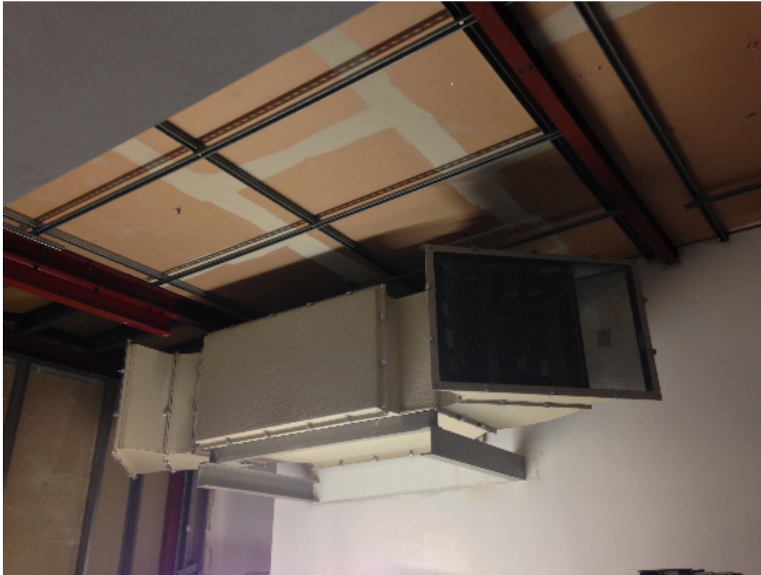
Figure 11: Smoke and heat exhaust ventilation system
