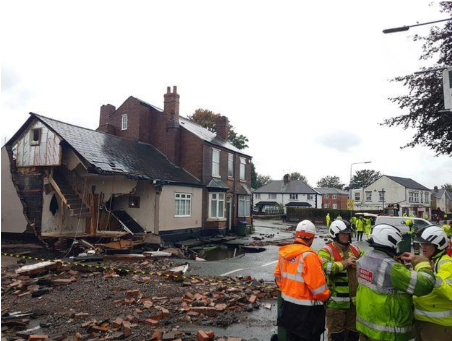
Figure: Image of a building damaged by a water mains failure, courtesy of West Midlands Fire Service
