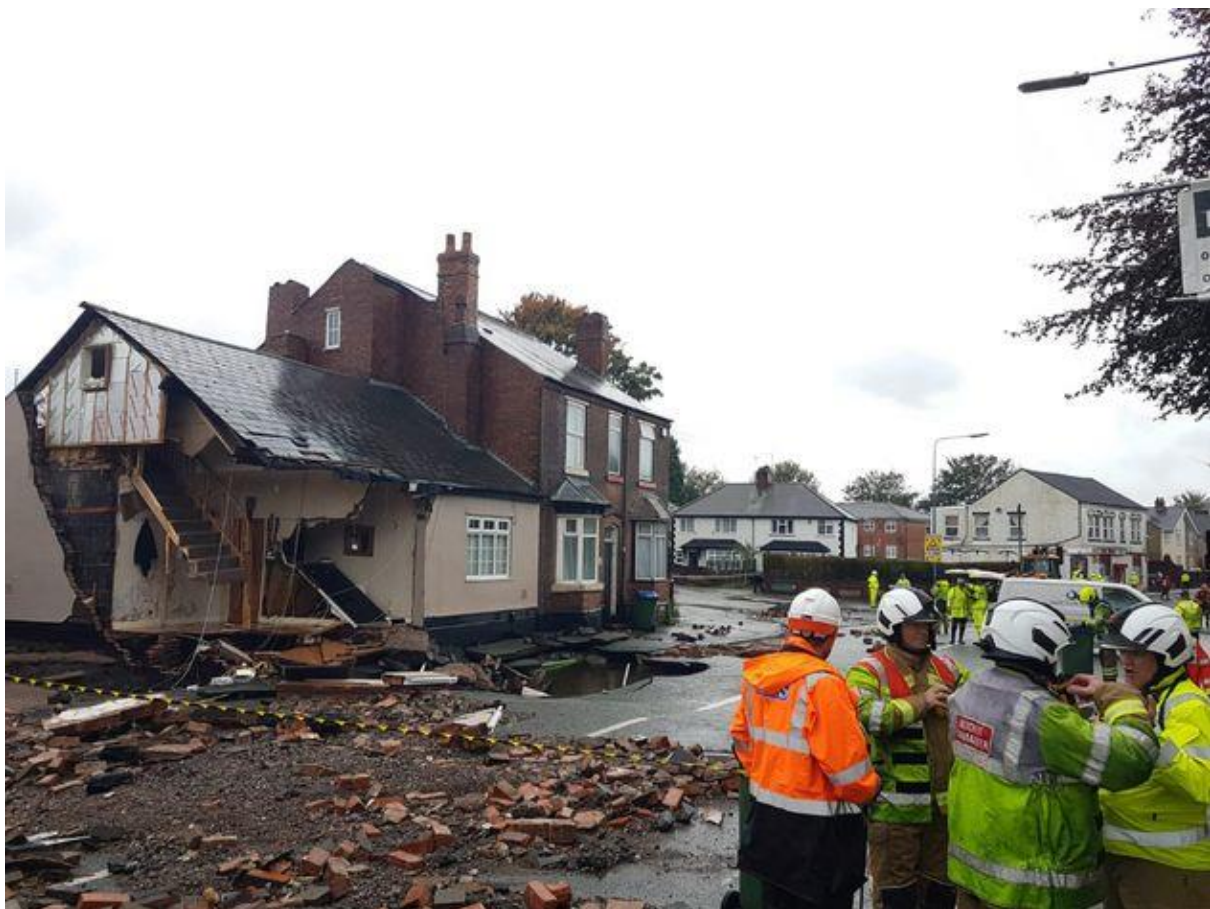
147 Figure: Image of a building damaged by a water mains failure, courtesy of West Midlands Fire 148 Service
