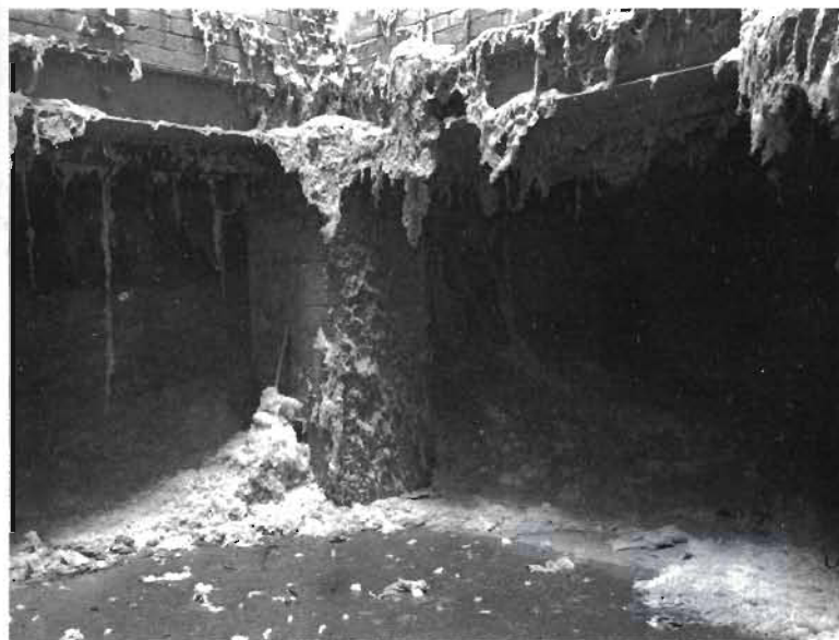
Plate 16. The base of a dust chamber in a cotton mill, where cotton dust and fly is collected by means of pneumatic trunking from the various machines. Fires often spread to the dust tower through the trunking. (Section 4).
