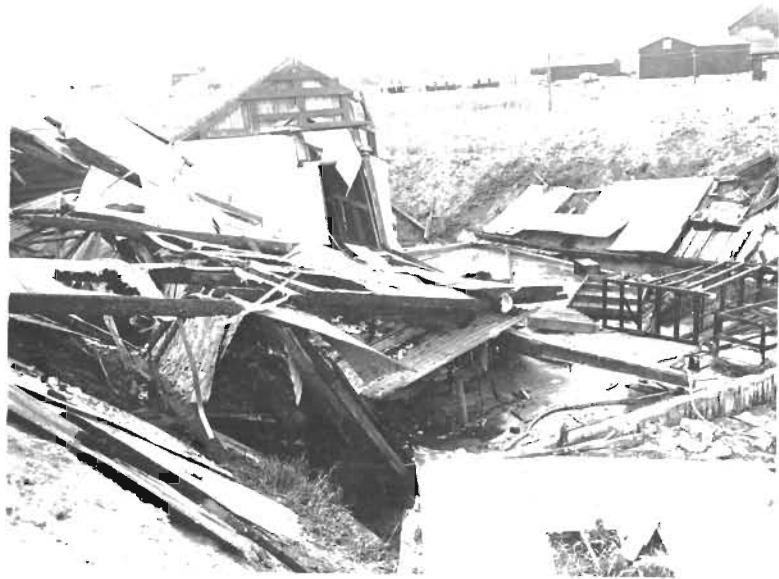
Plate 2. Complete devastation of a building in which nitro-cotton blocks were being dried, resulting in the deaths of three people. Note the earthworks round the building. (Section 2).
