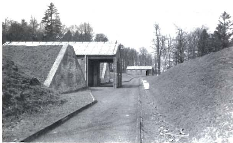
Plate 3. The earth traverse round this small explosive storehouse has the sides sloping at the natural angle of rest. The building in the background is untraversed. (Section 2).
