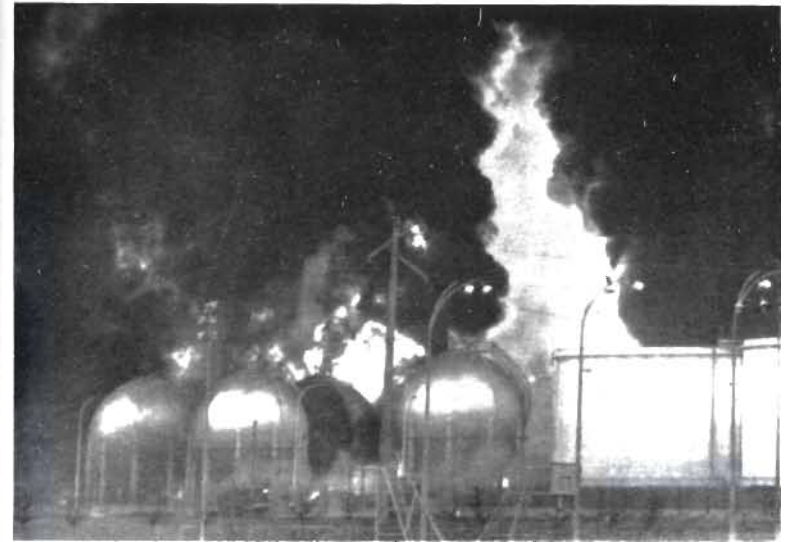
Plate 27. Fire resulting from an explosion at Feyzin refinery, near Lyon, France, where liquefied petroleum gas storage tanks were involved. 75 people were taken to hospital suffering from burns. (Section 5).
