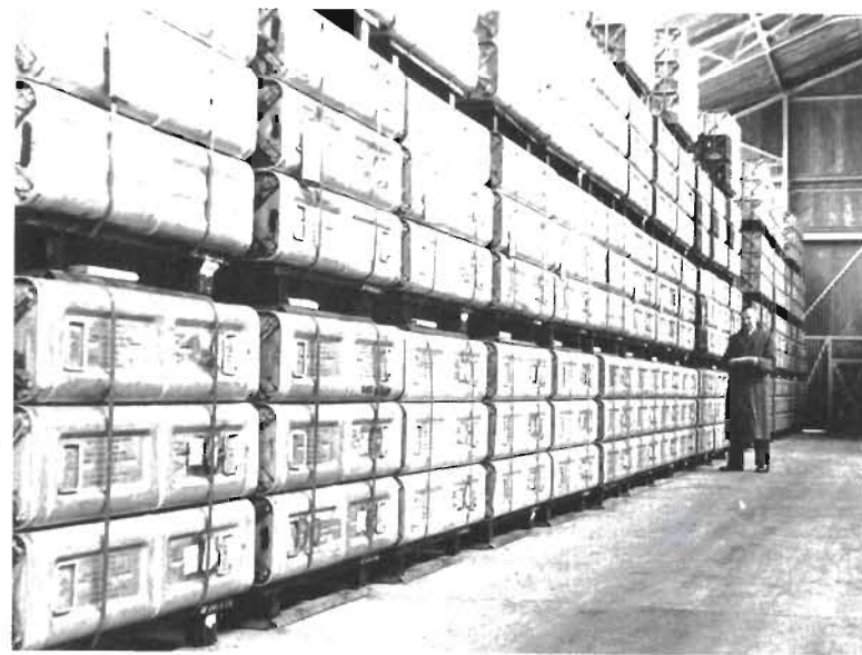
Plate 4. Interior of an explosives storehouse showing one method of storing ammunition by assembling it on pallets in 'unit loads'. (Section 2).
