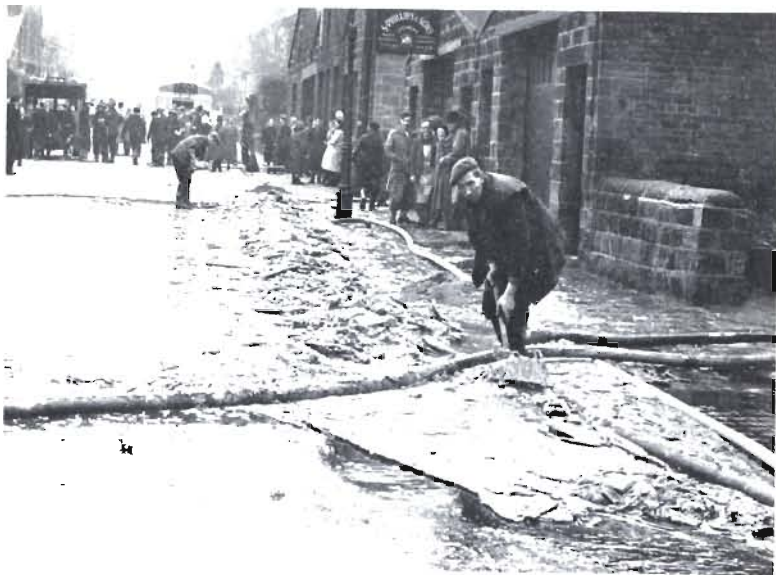
Plate 7. Paraffin wax solidified by water from branches after flowing from a fire. This caused considerable inconvenience by blocking the drains. (Section 3).
