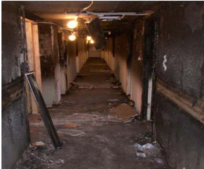
Figure 3 - Extended Length Corridor
