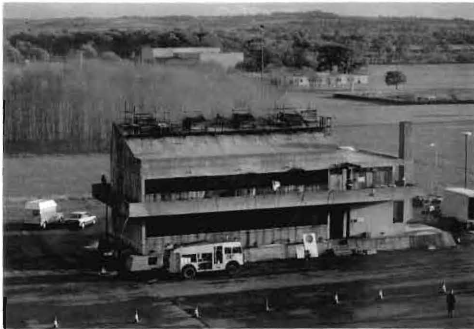
Figure 2: Industrial B building from the north-west
