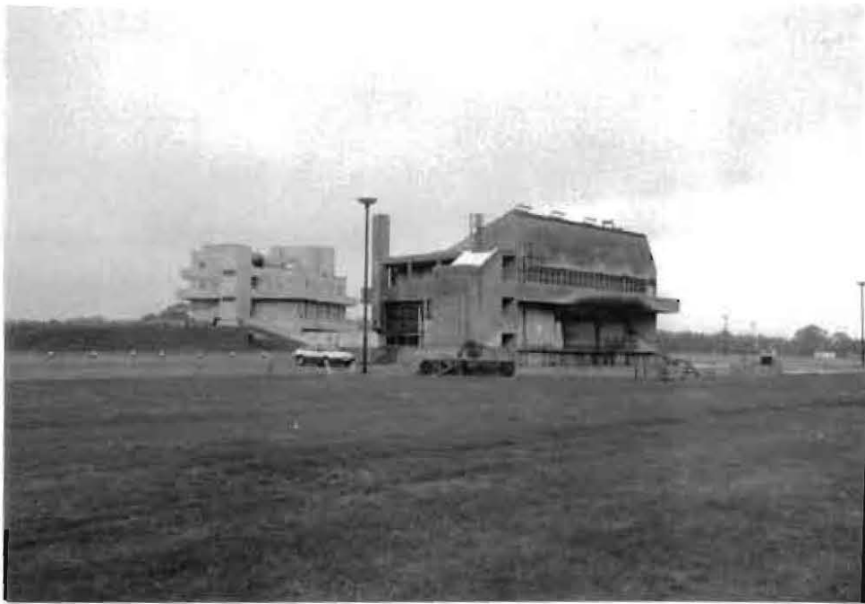
Figure 1: Industrial B building from the south-east
