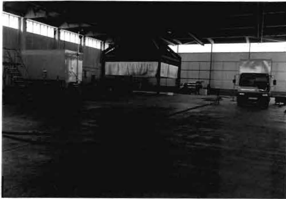
Figure 1 : The smoke hood in the Still Air Facility at RAF Little Rissington
