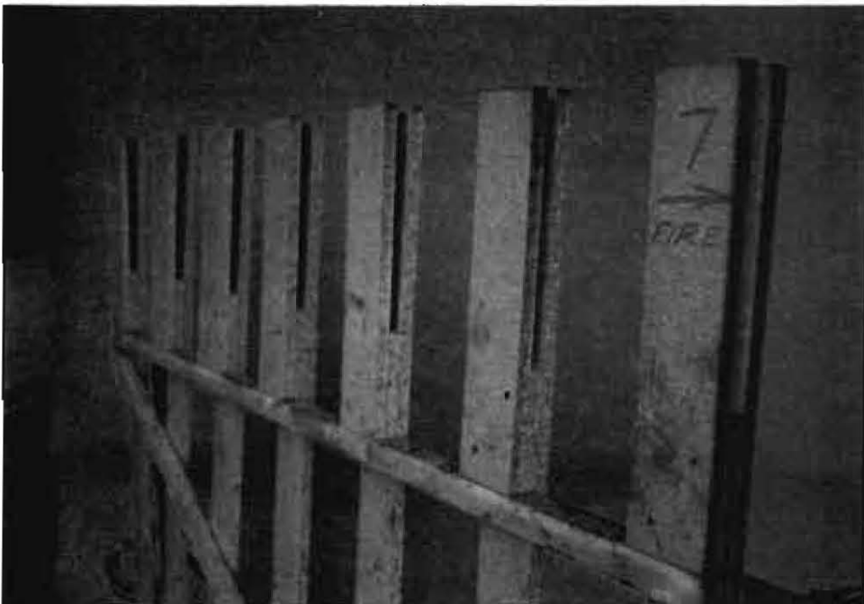
Figure 23 Fire Spread Witness Marks for Day 2 Test 3 (C222/1998)
