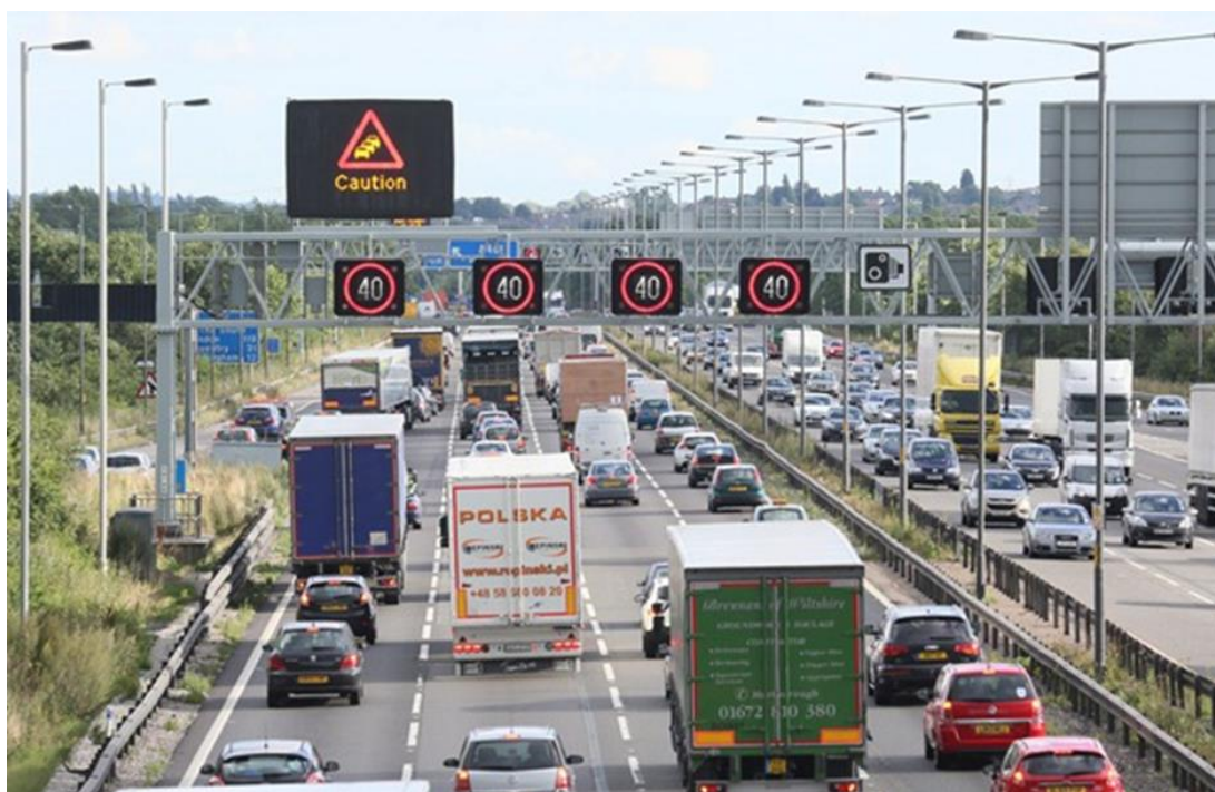
Figure 3-3: ALR motorway with lane signals showing queue protection
