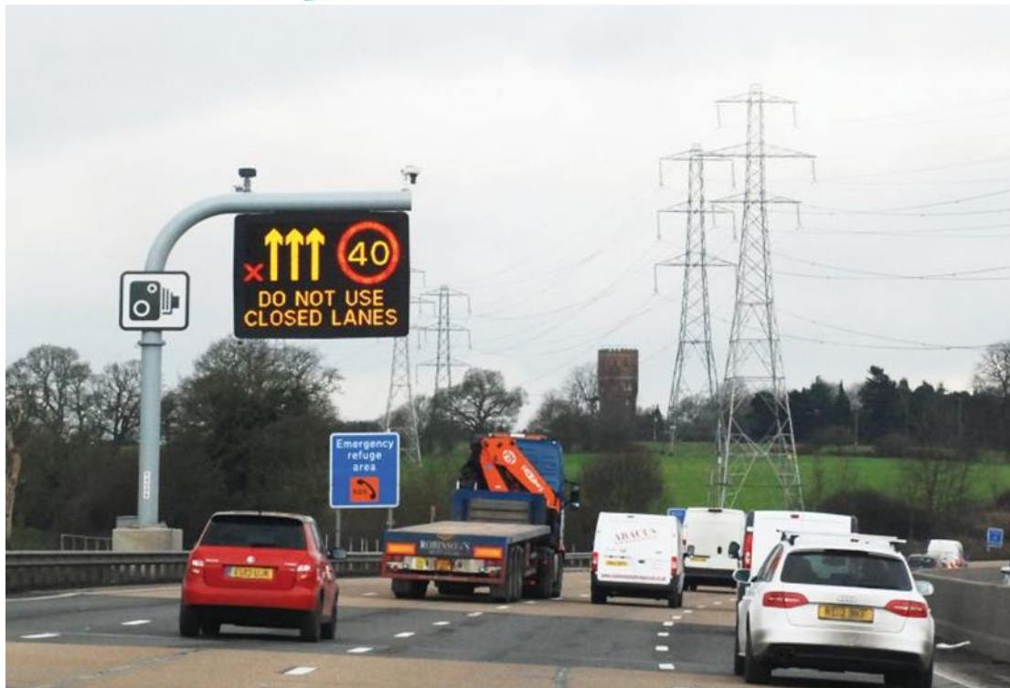
Figure 3-2: ALR motorway with a VMS showing lane 1 closed
